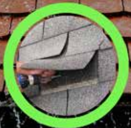
Roof Repairs & Replacements
