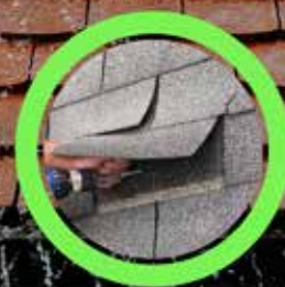
Roof Repairs & Replacements
